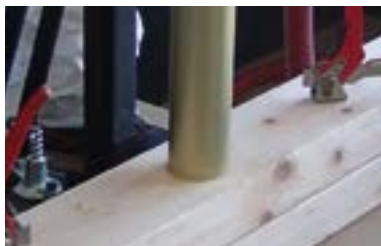
Trockenbohren in Holz
