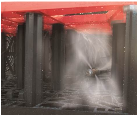
Jet washing the system
